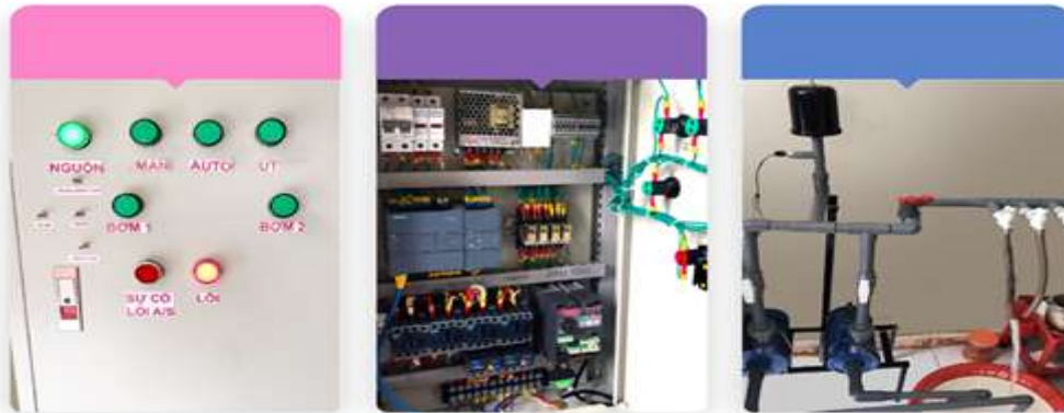
Figure 3.4: Finishing the control cabinet
